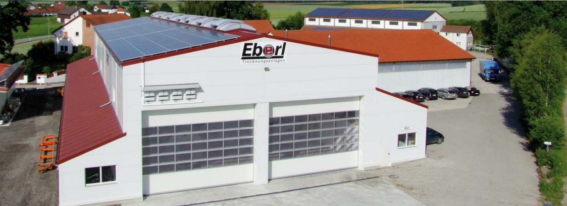
EBERL premises in Bodenkirchen, Bavaria / Southern Germany.
